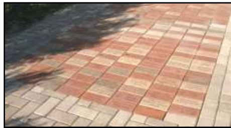
The new bricks that we ordered have been installed in front of City Hall.
