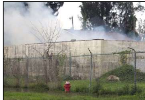
If you noticed smoke wafting over the north end of the City on Monday and Tuesday, it was a training burn conducted by our fire department to get rid of garden refuse collected by the City. The concrete block structure on the corner of Begonia and Camellia Streets is on the old power house premises which operated before LCEC took over our electricity supply in the mid 1950s.
