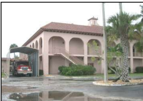
Ochopee Fire Control District opened a new station with a fire engine at Port of the Islands.
