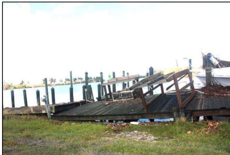
This and several other docks were lifted up or destroyed
