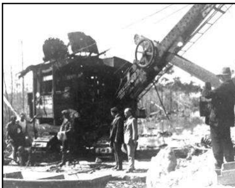
Excavation crew cr. 1926
