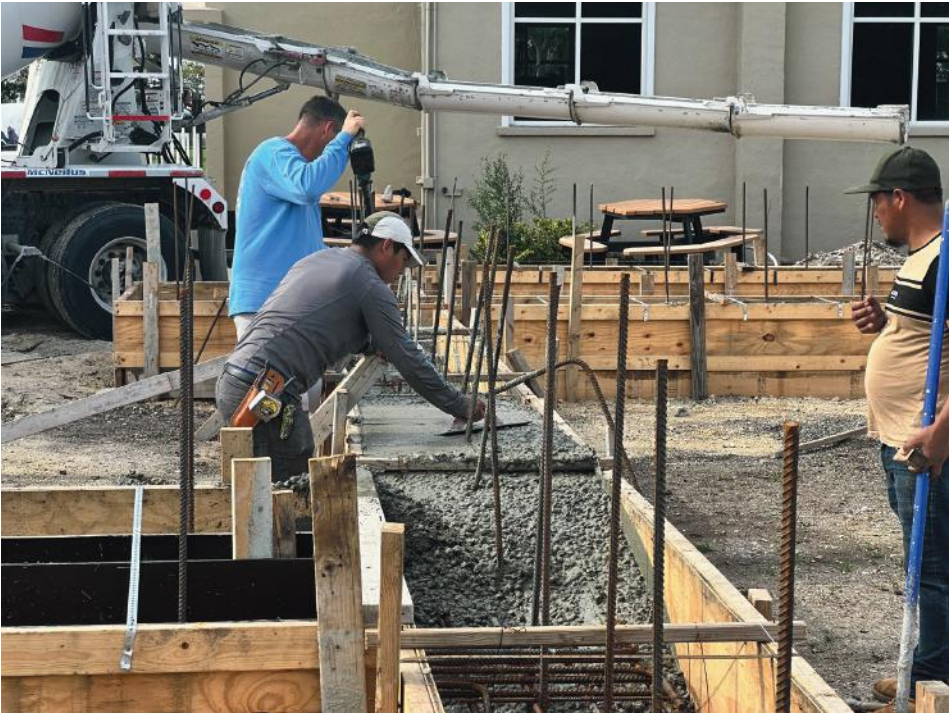
Pouring the foundation.
