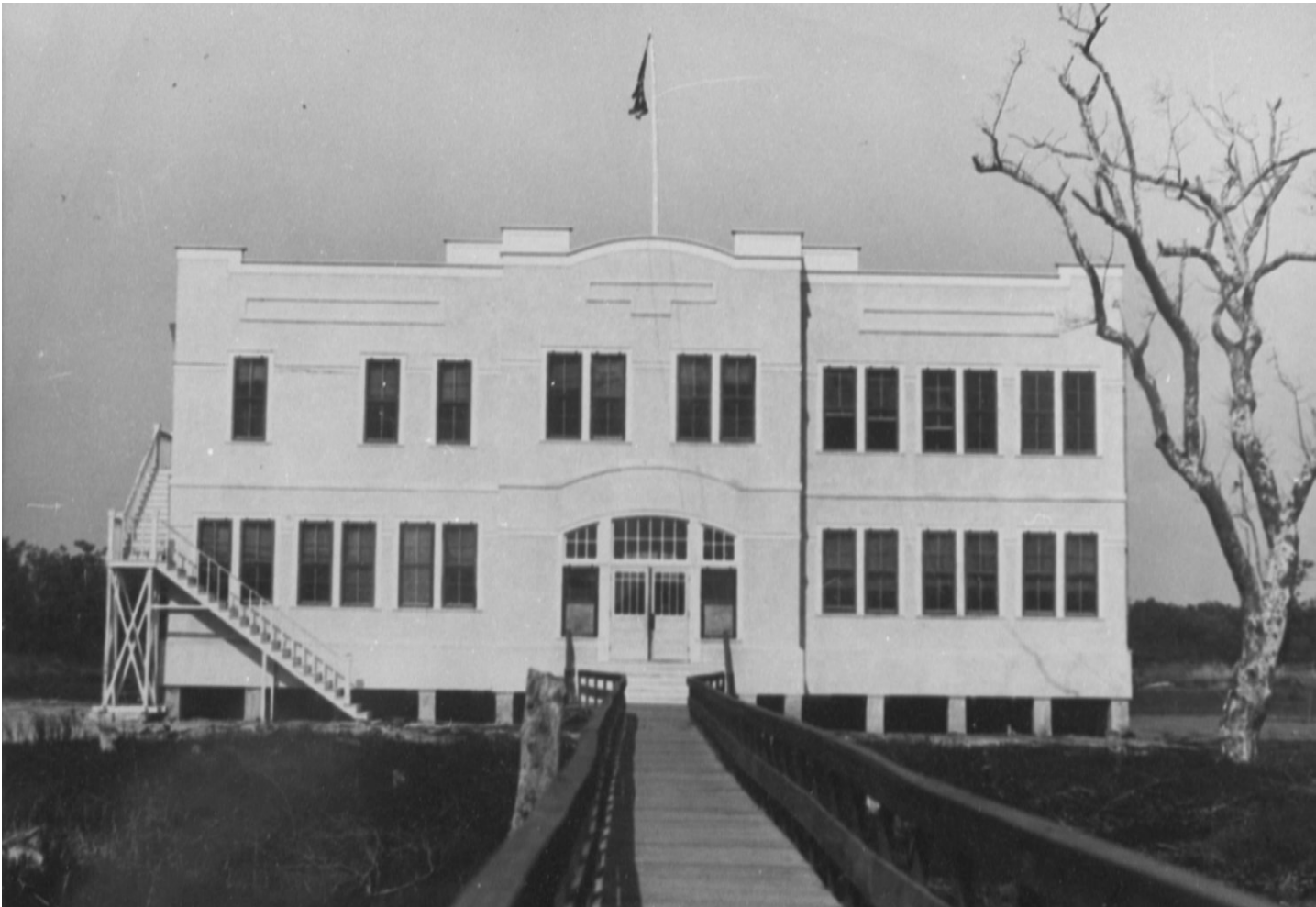
Photo Courtesy of Collier County Museums This is the original two-story building before it was torn down in the 1960s after Hurricane Donna. Collier County built new buildings in 1995-96 and completed the modern school campus serving pre-k through twelfth-grade students.
